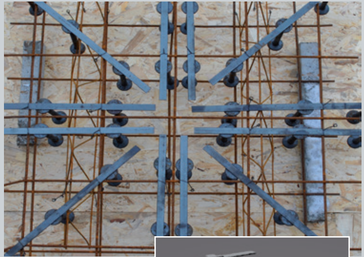
Figure 2 - Placement of Sheartech® rails
