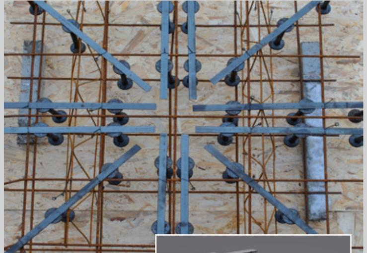
**Figure 2 - Placement of Sheartech® rails**
