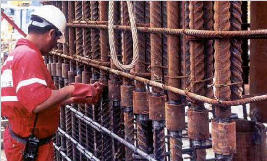
Bartec/Fortec couplers in diaphragm wall
