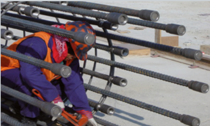
Bartec/Fortec couplers in pile cages
