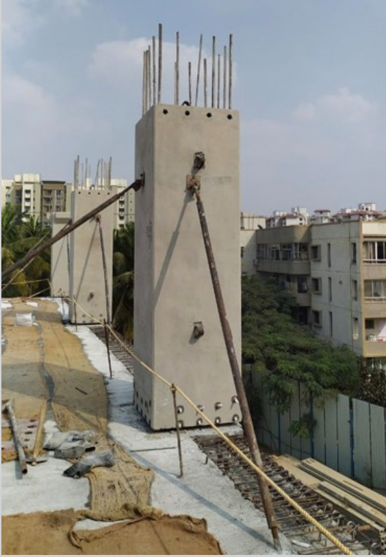
Groutec S Coupler in columns
