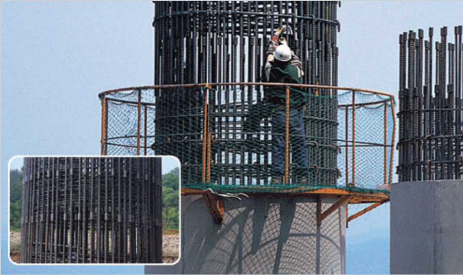
Construction of prefabricated rebar cage
