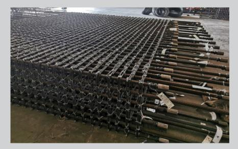
Prefabricated reinforcing bar cage for a core wall with 2 layers and staggered splice locations.
