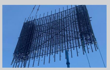
Prefabricated reinforcing bar cage using LENTON Ultimate PMO4 Hybrid Position Couplers being lifted into position for installation.
