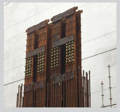
Weldable half couplers welded to structural steel columns.
