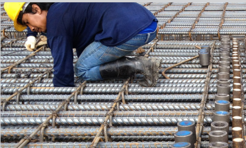
Bartec/Fortec R couplers in columns.
