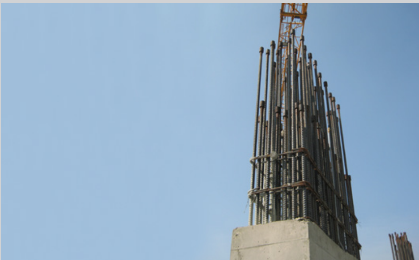
Bartec/Fortec R couplers in diaphragm wall.
