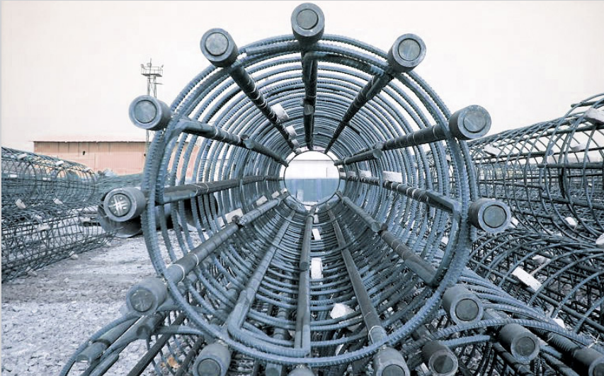
Bartec/Fortec R couplers in pile cages.
