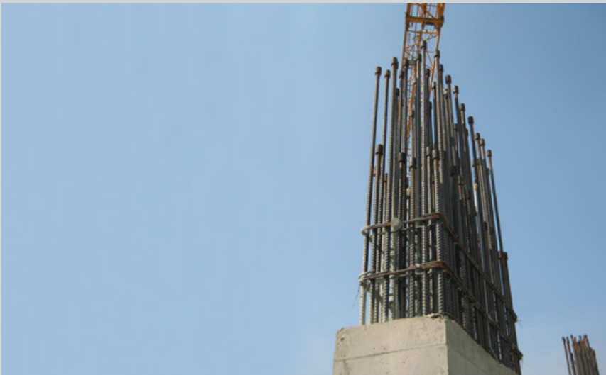
Bartec/Fortec couplers in diaphragm wall.
