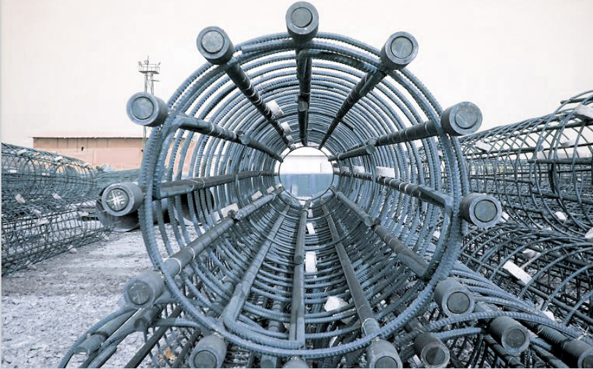
Bartec/Fortec couplers in pile cages.
